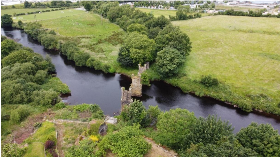
Figure 3-6 - River Finn Railway Bridge piers
