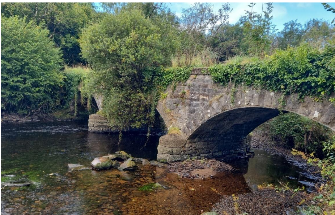
Figure 3-7 - Masonry arch bridge at Lough Eske
